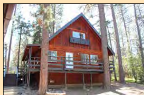
HEAD TO TOE REMODEL! Tile and granite + new flooring. 3 BR, 1-3/4 BA, 1600 sq.ft., oversized garage and ART STUDIO. Fenced, on sewer, walk to town. MLS#2008158 $375,000
